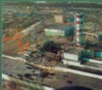
Chernobyl Nuclear Power Plant.
